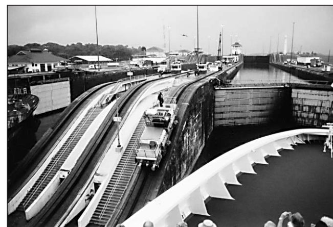
It takes about nine hours for a large cruise ship to transit the canal. Tugboats aid the ship's entry into the locks from the Atlantic Ocean. Tiny train engines, called "mules," run along the shore to help guide large ships through the canal.
