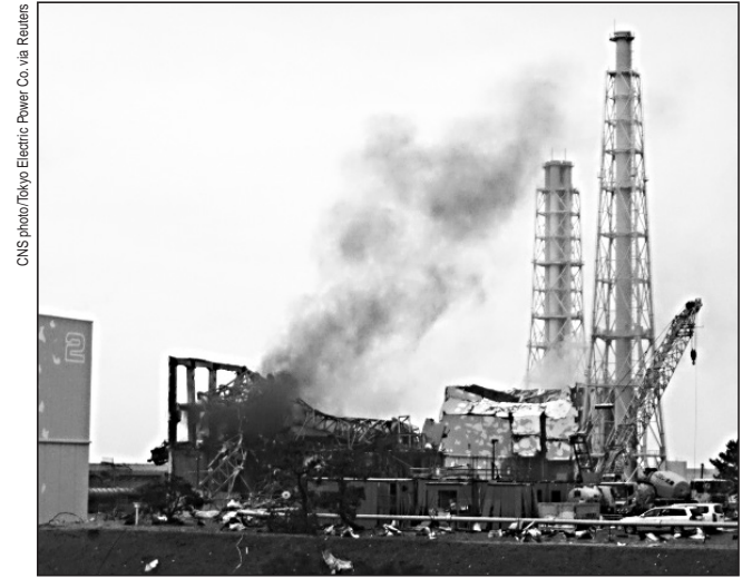
Smoke is seen coming from the area of the No. 3 reactor of the Fukushima Dai-ichi nuclear power plant in Tomioka, Fukushima prefecture, Japan, on March 21 in this handout photo from Tokyo Electric Power Co. Workers at the earthquake and tsunami damaged plant were evacuated after smoke was seen rising from the nuclear reactor.
